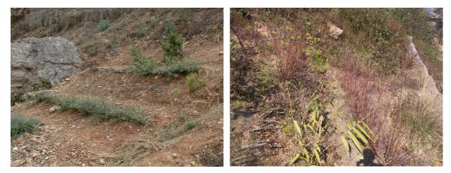
Fig. 9 The hedge brush layer construction shortly after completion (left)- 2001 and about one year later (right) –2002 in Thankot (Nepal)
