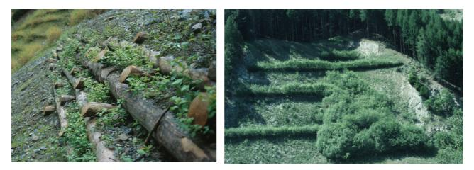
Fig. 6 A detail of a vegetated cribwall after 6 months (left)-1994 and after 4 years developing (right)-Suldenbach-1998
