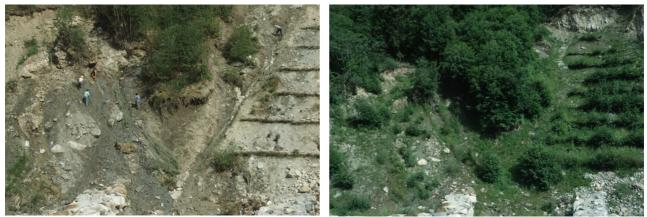
**Fig. 5** Overview of the project area Suldenbach (Italy) beginning with the implementation of drain fascines (left)- 1990 and after developing 2 years (right) - 1992
