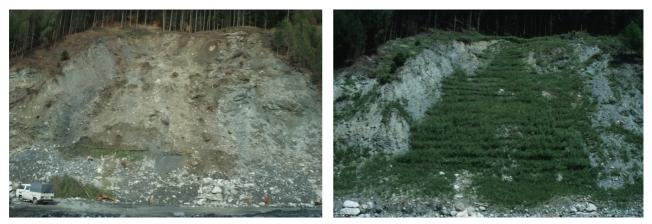
Fig. 4 Overview of the project area Suldenbach (Italy) beginning with the implementation of hedge brush layers (left)-1989 and after developing 3 years (right) - 1992
