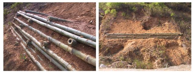
Fig. 10 Vegetated bamboo cribwall constructed in Thankot (Nepal)- 2002
