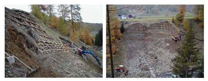
Fig. 7 Construction of a vegetated slope grid based on a vegetated cribwall - Karlinbach 2001
